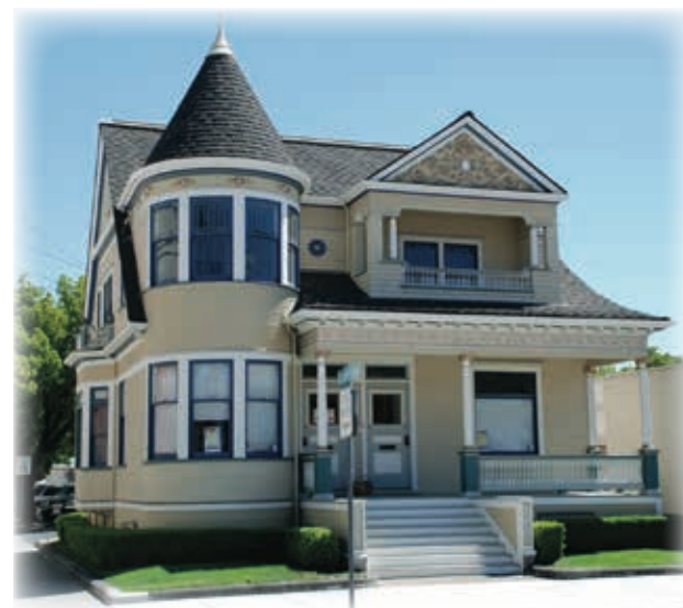
(In Historical Downtown Gilroy off Monterey Street)
